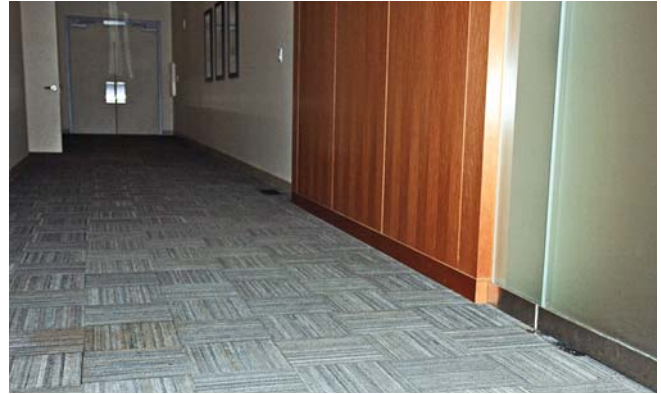
Tire Tile Hallways — Recycled aircraft tires molded into squares create an ideal flooring for high-traffic areas.
