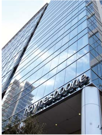
Haynes and Boone has moved into One Victory Park in Dallas, a LEED-certified Silver core-and-shell building.
